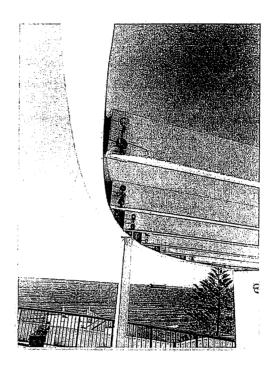
Some of the bolts holding up the rooftop pergolas are very rusty, Programmed proposes to replace these rusted bolts with stainless steel bolts to prevent any further corrosion & damage.
