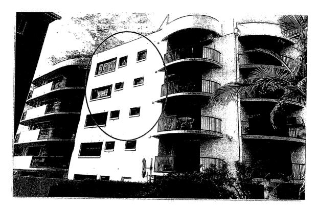
The top six meters of the sheer wall on the right side of the building is showing signs of water damage & cracking, Programmed will grind back any loose & flaky paint, sika-flex any cracks, seal the top half of the wall with a penetrative sealer/ binder ( to help with adhesion), then paint the wall with two coats of high quality flexible exterior paint ( same as the rest of the building).
