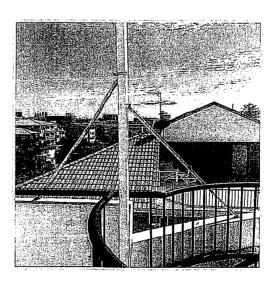
The T.V. antenna bracket, Foxtel dish bracket & the pipe brackets are also extremely rusty & are in need of replacing.
