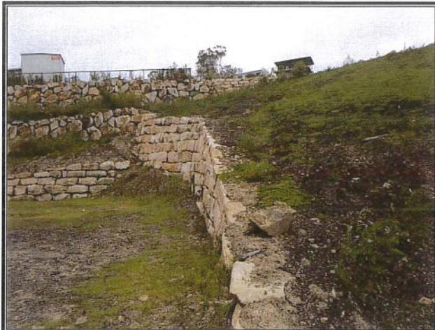
Existing rock retaining walls
